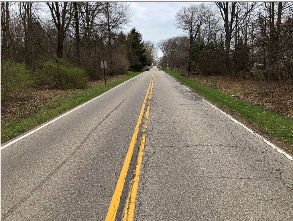
Picture 4 – Sunnyside Road looking north approx. 375' south of Shady Lake Drive. Several longitudinal cracks adjacent to centerline. Wheel track and edge cracking is prevalent, areas of base failure.
