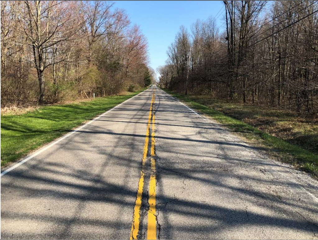
Picture 3 – Sunnyside Road looking north approx. 2,000' north of the Norfolk Southern railroad tracks. Pavement centerline joint is separated, with additional longitudinal cracking adjacent to centerline. Asphalt pavement has been patched along edges.
