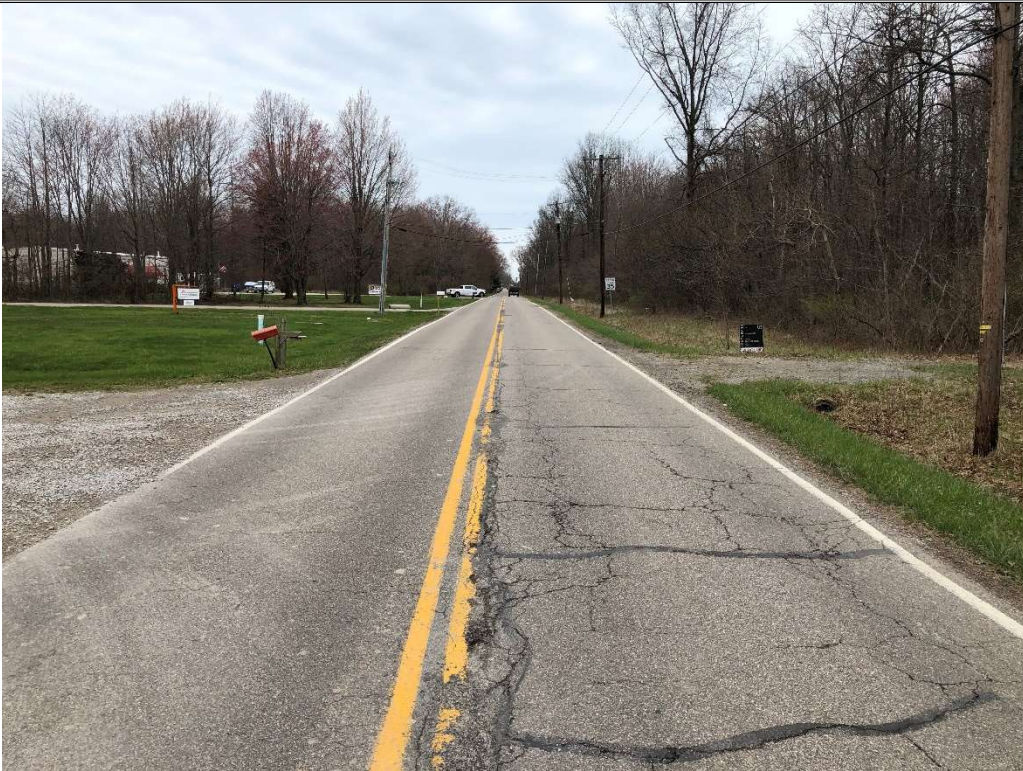
Picture 2 – Sunnyside Road looking north approx. 1,400' north of the Norfolk Southern railroad tracks. Pavement centerline joint is separated and temporary patching has debonded in areas. Map and wheel path cracking.
