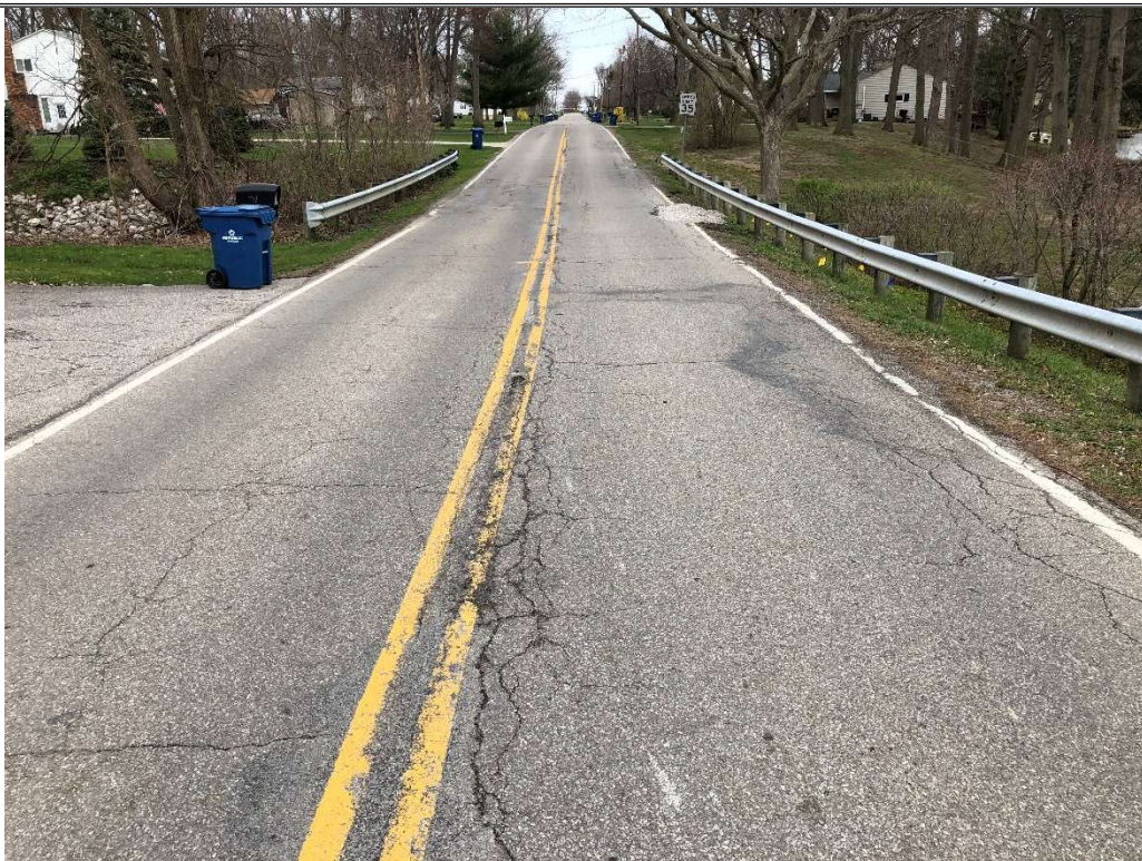
Picture 6 – Sunnyside Road looking north, just north of Shady Lake Drive. Pavement above the existing culvert is in poor condition. Pavement base is exposed on northbound lane and southbound lane has large asphalt patching areas. Guardrail is noncompliant in height and end assemblies.
