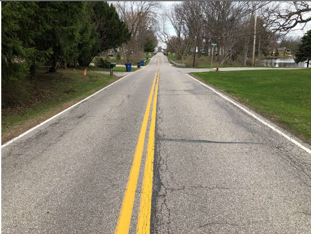
Picture 5 – Sunnyside Road looking north, just south of Shady Lake Drive. Longitudinal cracking along centerline. Pavement has delaminated in areas of the wheel track cracking and withing patched pavement areas.
