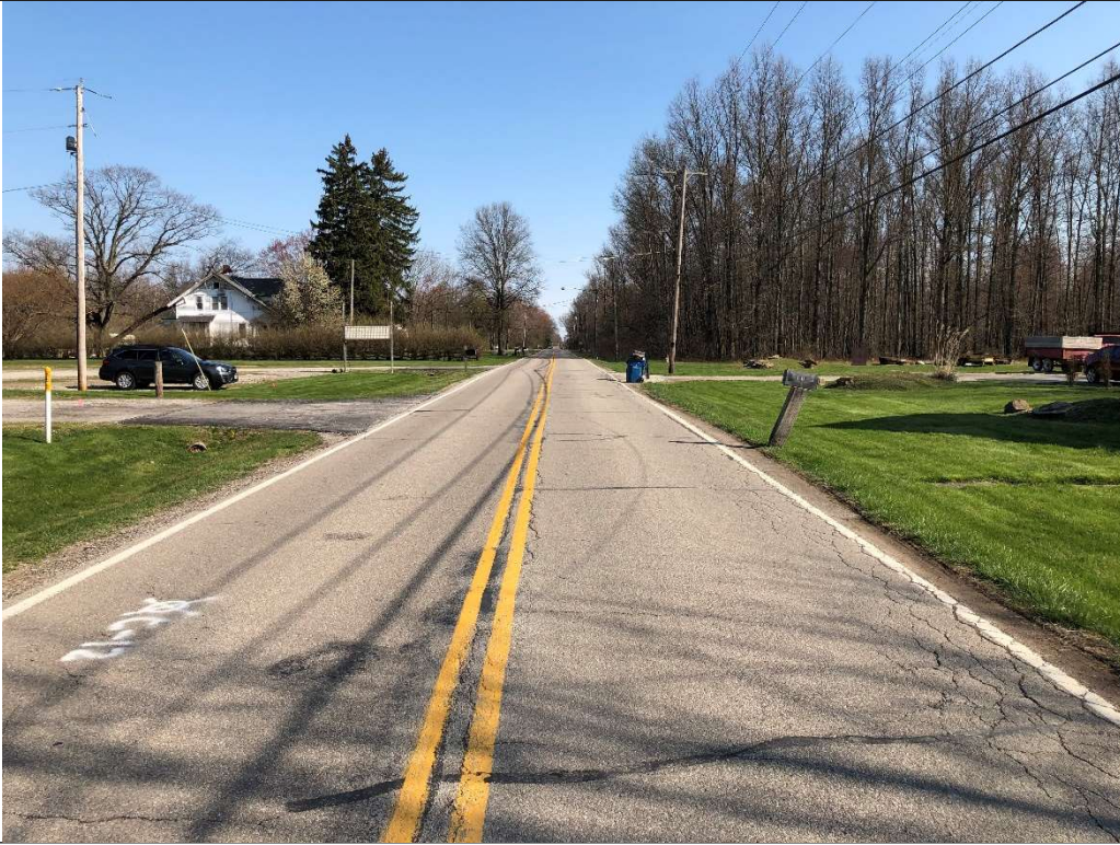
Picture 1 – Sunnyside Road looking north approx. 800' north of the Norfolk Southern railroad tracks. Longitudinal pavement joint cracking and wheel lane/edge cracking on outside of northbound lane.
